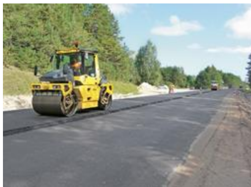
Fig. 7. BW 174 AP (10 t) equipped with BCM net
